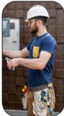
Electrical, Mechanical & Plumbing (MEP)
